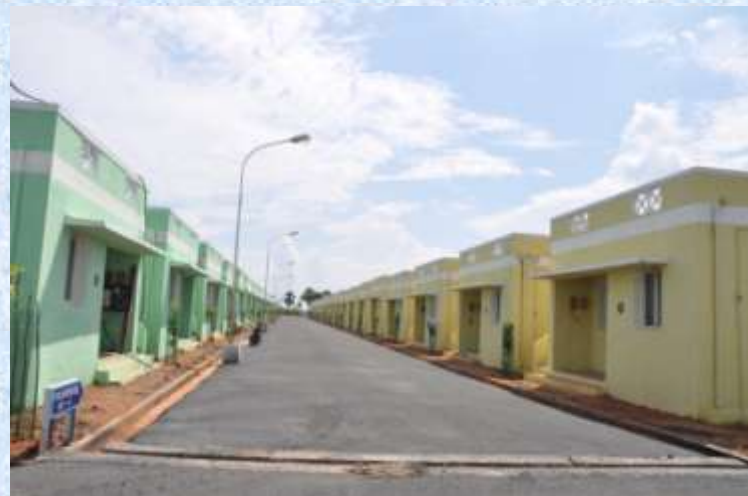
Under PIA, Tsunami houses was constructed a cost of Rs.21 crore in the Nallavadu Village, Puducherry
