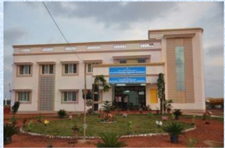
New Regional Transport Office Complex was constructed at Karaikal .
