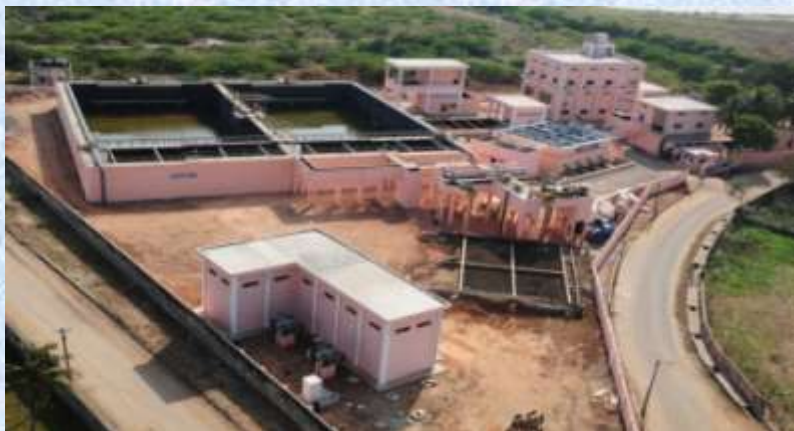
17 MLD Sewerage Treatment Plant at Dubrayapet at a cost of Rs.300.65 crore.
