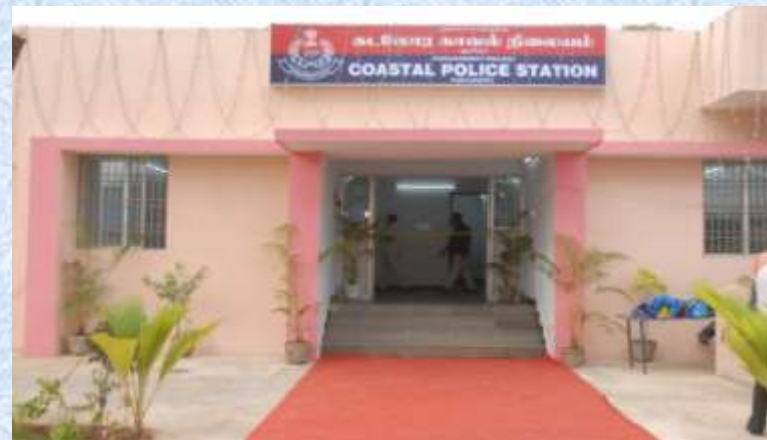
Coastal Police Station constructed at a cost of Rs.37.57 lakh in the Thengaihittu Fishing Harbour
