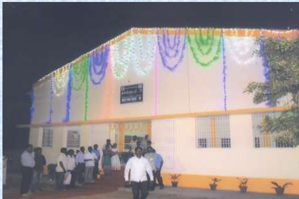
Two Rural Godowns was constructed in the premises of Karaikal Market Committee.
