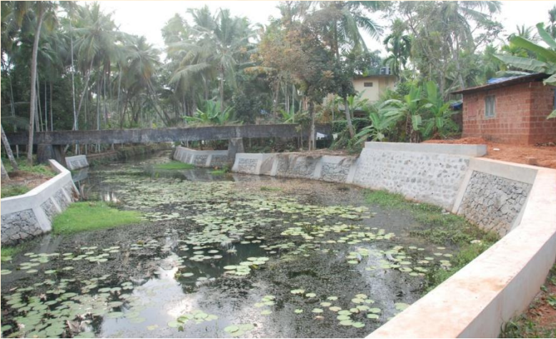
Construction of retaining wall from Ayyappankavu Pandakkal to Moolakkadavu bridge
