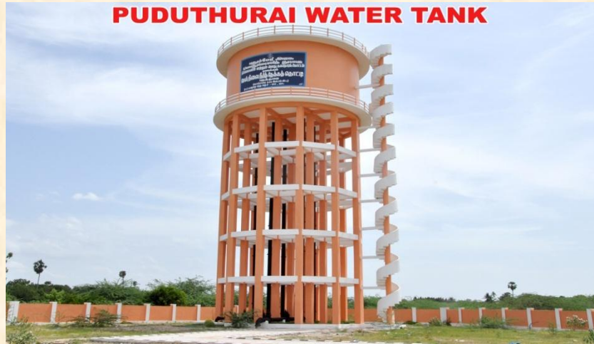
Water Tank at Puduchurai, Karaikal
