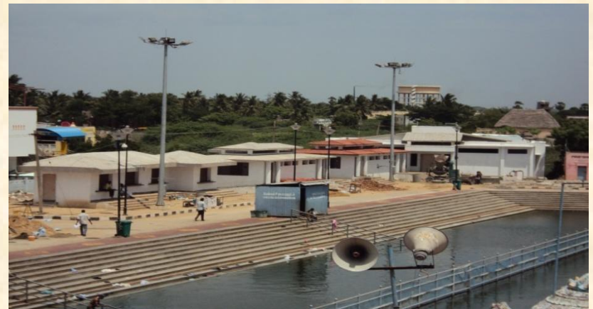
Toilet Block at Nalan Kulam, Thirunallar
