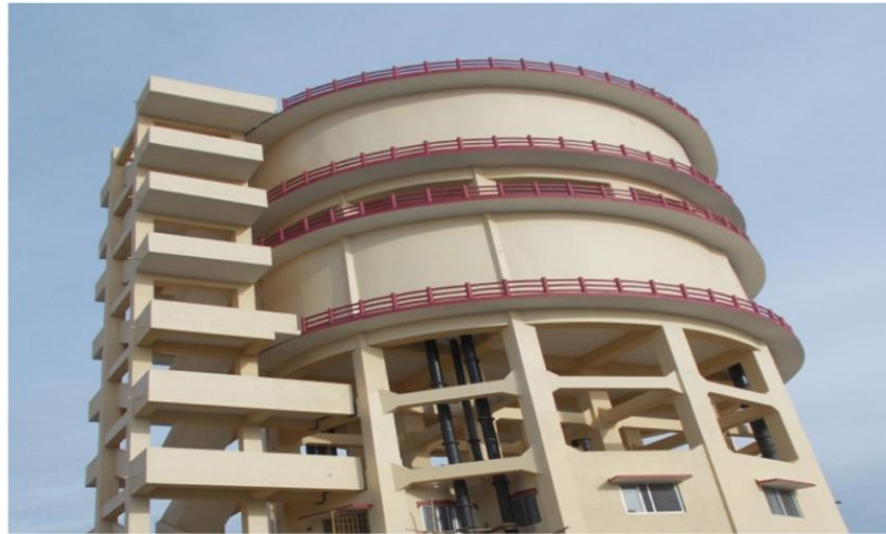
Over Head Tank at Thanthai Periyar Nagar
