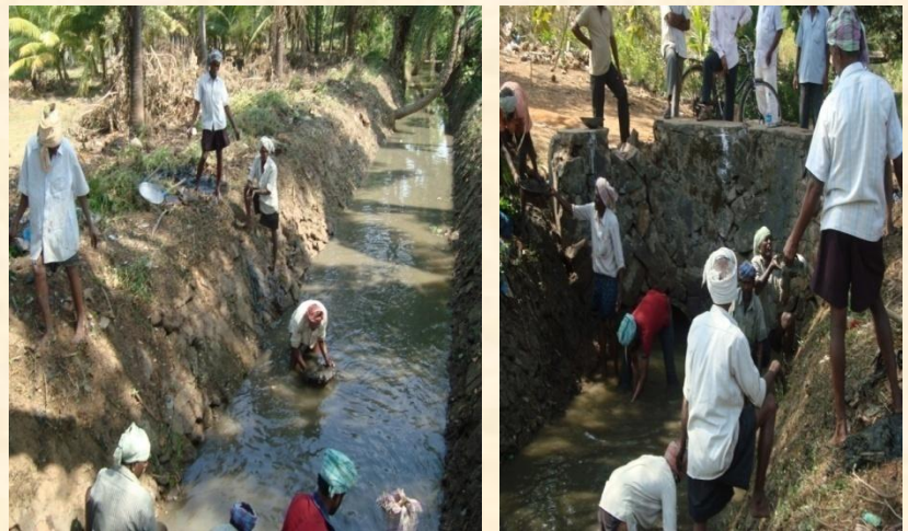
Desilting the Irrigation channels
