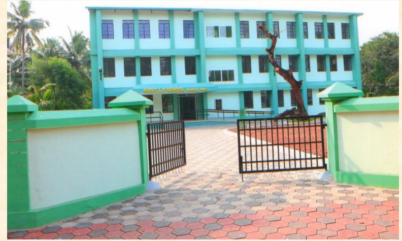
Newly constructed Govt. L.P. School, Parakkal.
