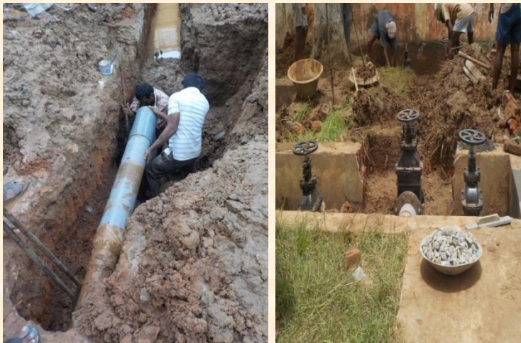
Improvement to the water supply system at Kanakalapeta
