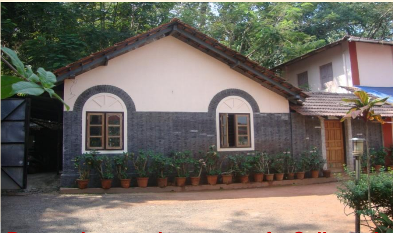
Renovation and reuse of Collector's Bungalow
