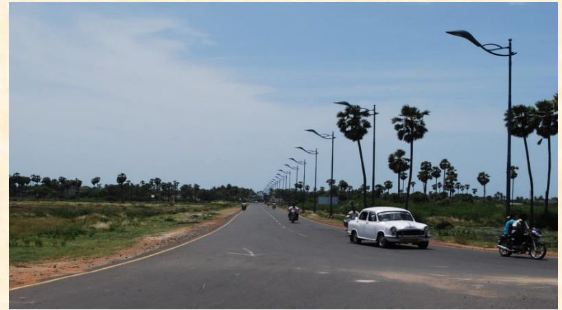
Laying of FCI Road, Near Bus-stand
