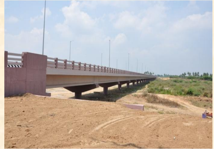
Manamedu Bridge, Puducherry
