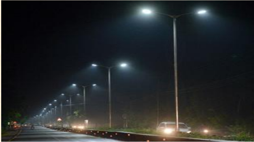
A view of LED Street Lights from Kanagachettykulam to Pillaichavady
